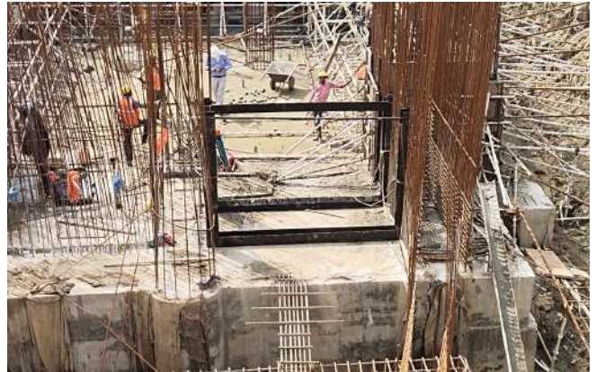
Stop Log Gates And Trash Rack Screens Erection Work at Site
