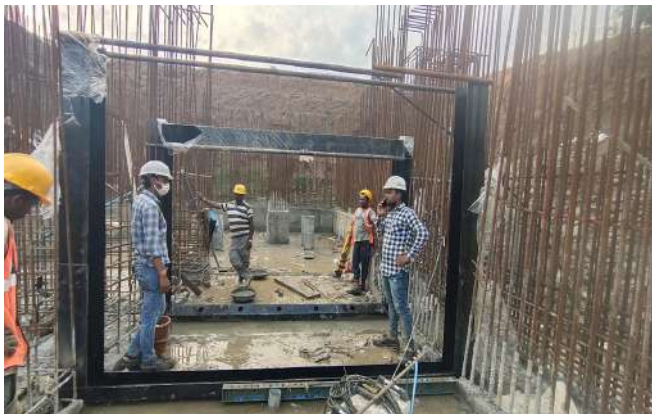
Stop Log Gates And Trash Rack Screens Erection Work at Site
